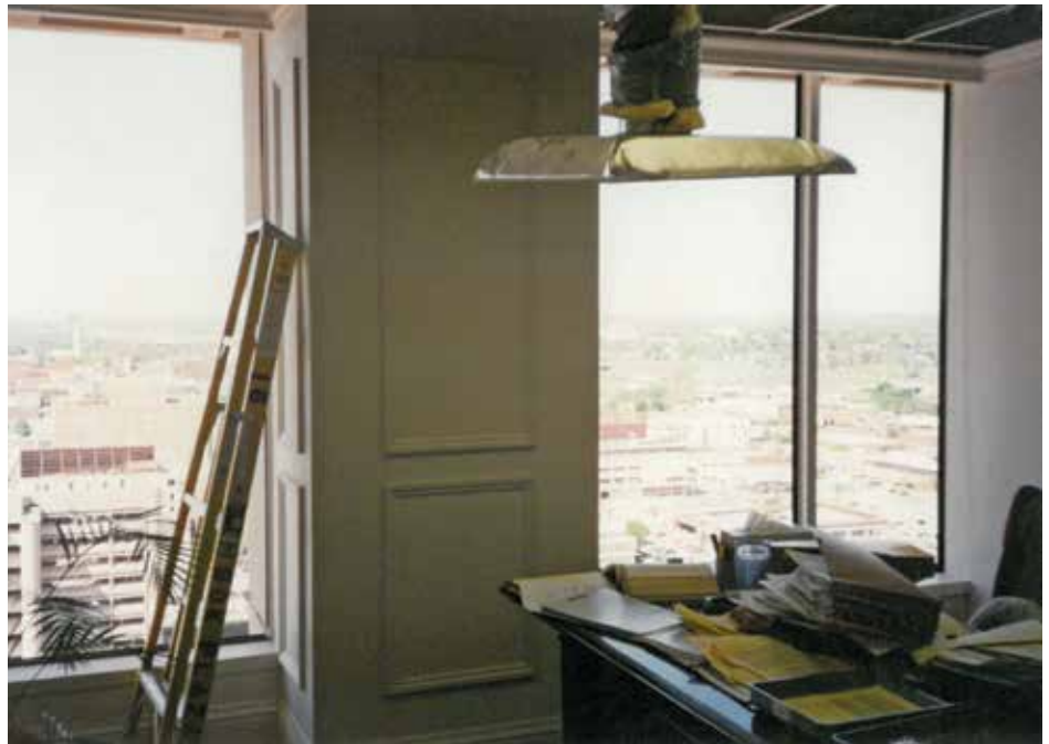
Located two blocks from the Murrah Building, windows were blown out of Susan's office. Light fixtures and ceiling tiles also fell as a result of the bomb's blast.
