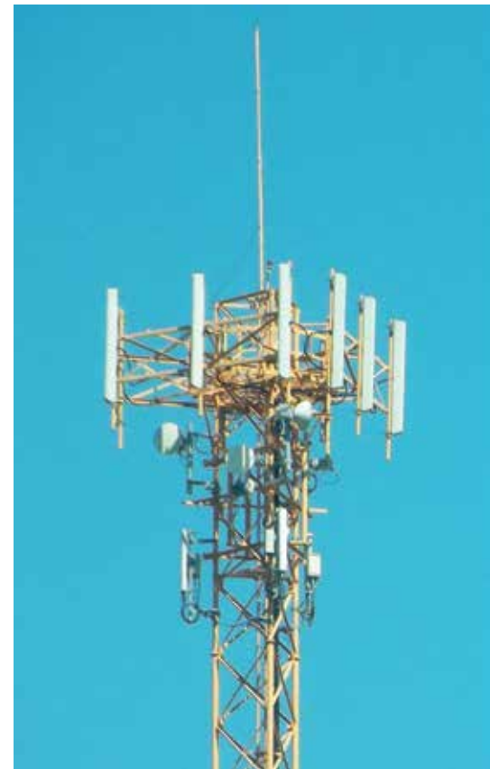
Figure 1: Cell site with 3 sectors
